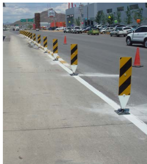
Figs 10 & 11. When the trails are located within the Clark St. right-of-way, alternating lane markers (left) and flexible hazard markers (right) will separate the trails from the adjacent traffic lane as shown above.
