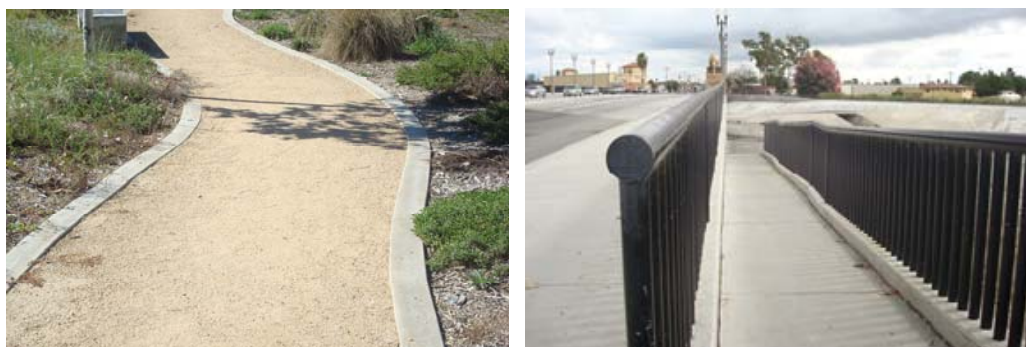
Fig. 3 & 4. A decomposed granite path with concrete curbs and concrete ramp with metal railings. Design to match depicted ramp.
