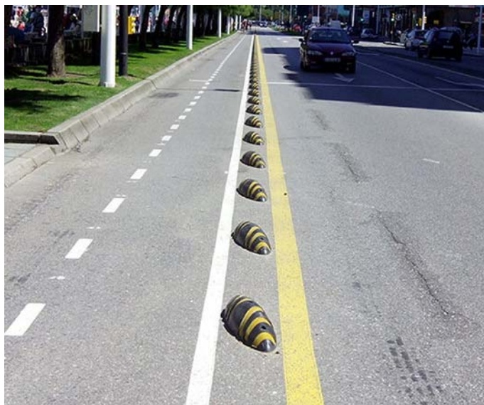
Figs 10 & 11. When the trails are located within the Clark St. right-of-way, alternating lane markers (left) and flexible hazard markers (right) will separate the trails from the adjacent traffic lane as shown above.
