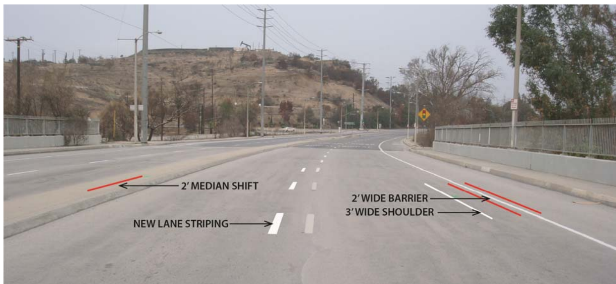
Fig. 5. San Gabriel Blvd Bridge with striping and median changes to accommodate the Class IV Bikeway
