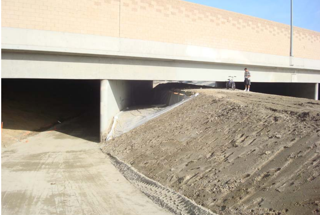
Fig. 7. Example of west side underpass improvements including de-watering site along the Rio Hondo at the Interstate 10 Freeway . Similar improvements for the implementation of the trail at the Rosemead underpass are necessary for trail accessibility and continuity.
