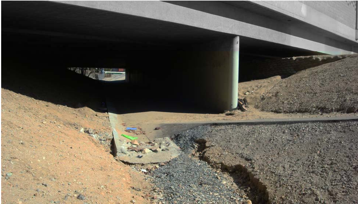
Fig. 5. Recently renovated underpass with new concrete V-ditch.
