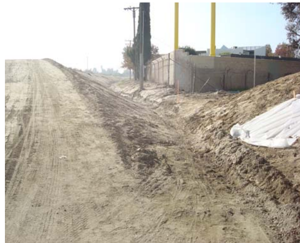
Fig. 4. The recently constructed drainage channel in the hiking and riding easement, looking southwest.
